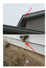
24. Gas Meter: I noticed the smell of gas every time I walked near the gas meter. The gas meter was being pulled downward by the settling concrete at the rear service door. The concrete should be carefully removed and then the gas meter and piping should be carefully checked for leaks. This needs correction as it is a hazard. If the concrete is to be re-installed, the pad should be smaller, and should not be poured around the gas piping.
