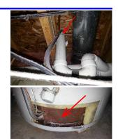
I was not able to open the cover to light the pilot light, because it was rusted closed.
